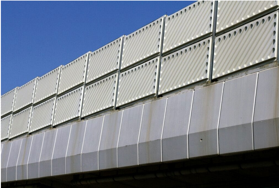
Figure 18. Tyre-based noise walls (Roadline, 2022).
